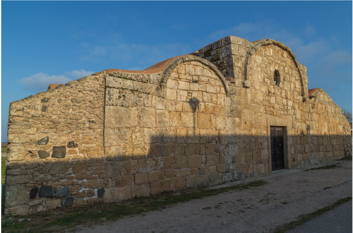
Fig. 51 - Façade of the church of San Giovanni (photo by Unicity S.p.A.)
