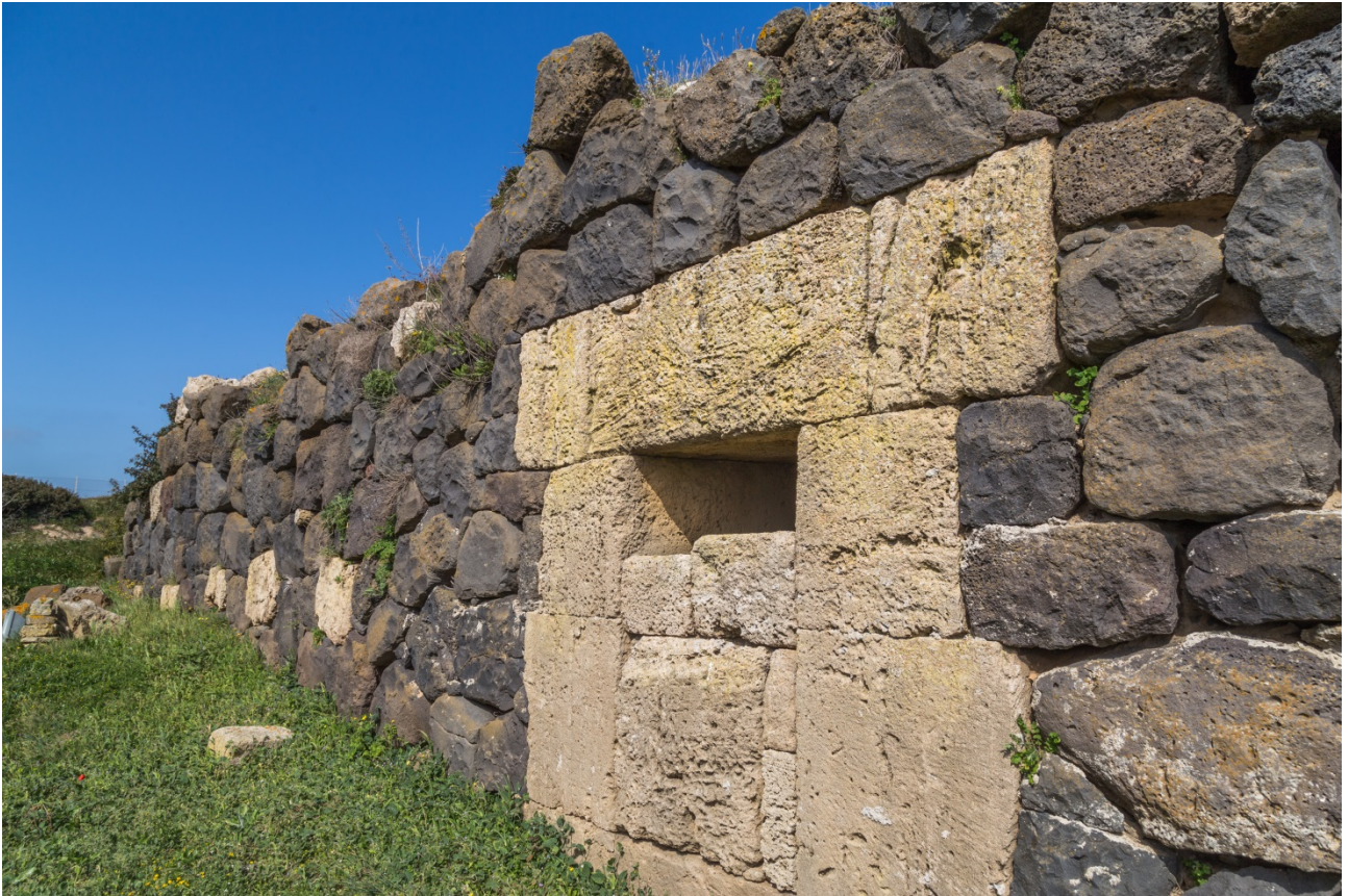
Fig. 10 - The Punic wall with the postern blocked up during the Roman Era (photo by Unicity S.p.A.)
