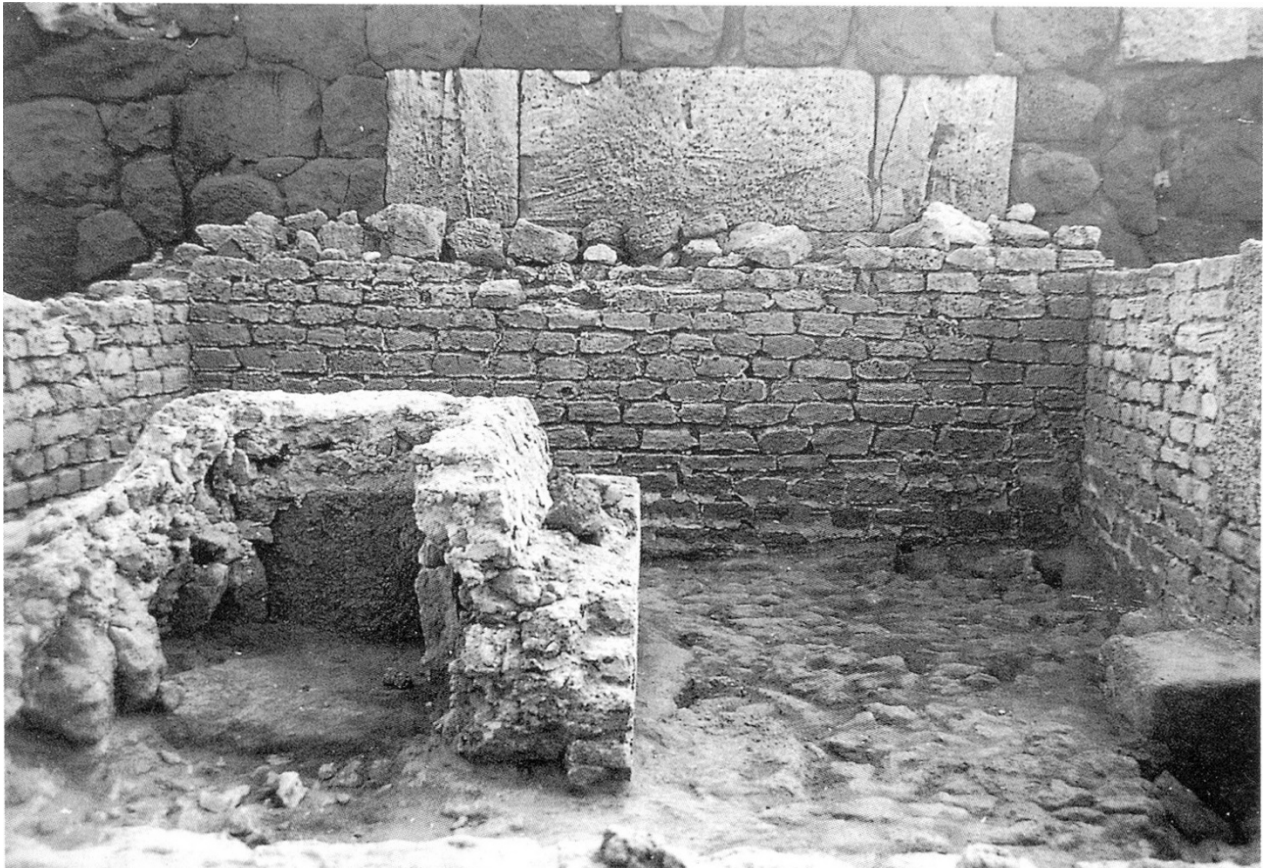
Fig. 12 - The funeral chamber in the moat, that blocked the postern in the walls (photo C. Tronchetti)
