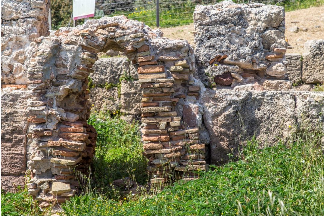
Fig. 30 - Thermal baths nr. 1: the entrance to a praefurnium (photo by Unicity S.p.A.)
