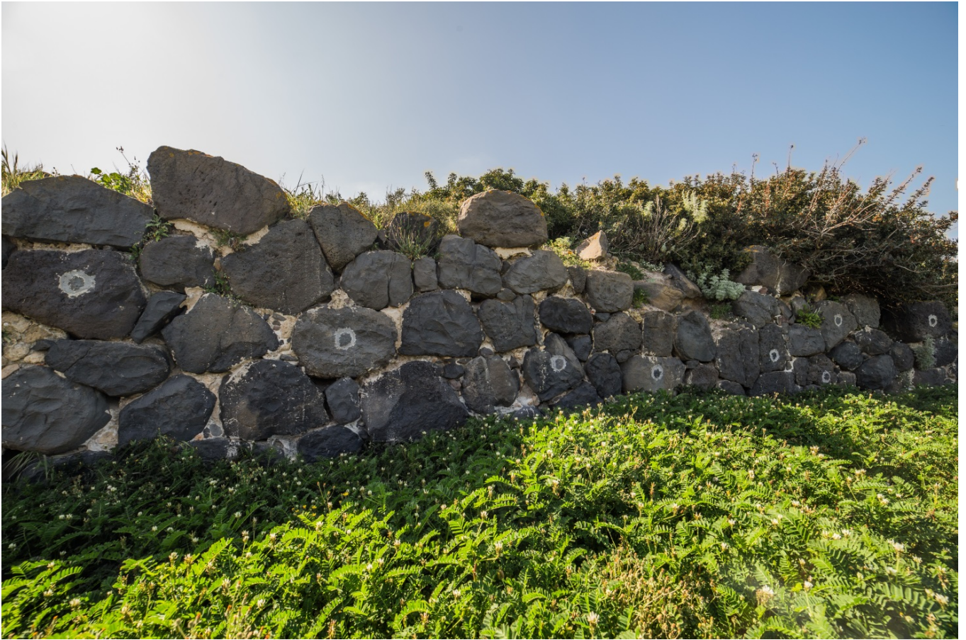
Fig. 11 - The moat's counterscarp wall (photo by Unicity S.p.A.)
