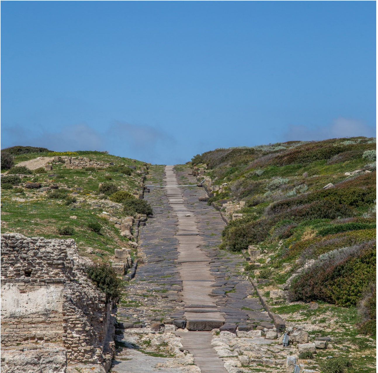
Fig. 16 - A road in the Roman city; the modern covering of the sewer in the centre (photo by Unicity S.p.A.)
