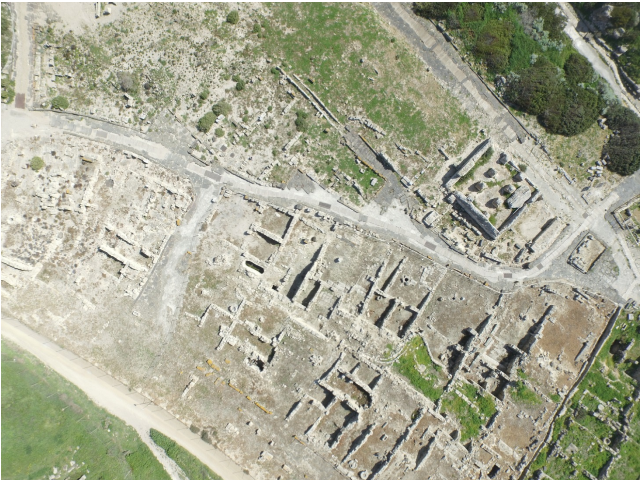
Fig. 40 - Roman houses on the slopes of San Giovanni hill, west of the castellum aquae (photo by Unicity S.p.A.)
